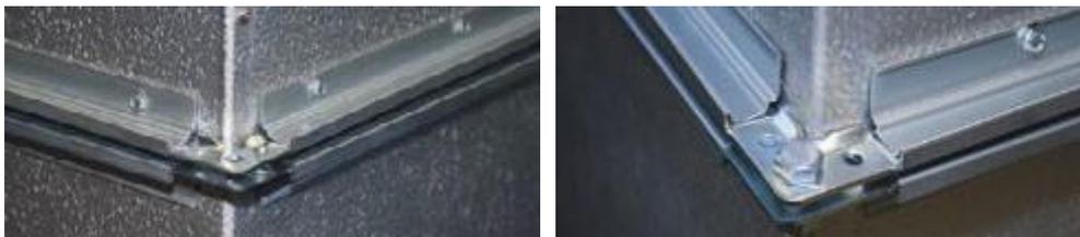
For extra watertightness, a stainless steel sliding strip is hammered onto the top of the DW profile. This should overlap the corner piece by at least 1.5 cm.
